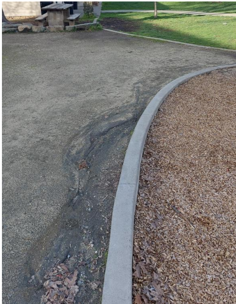
Figure 3: Erosion of DG around playground and behind Community Center
