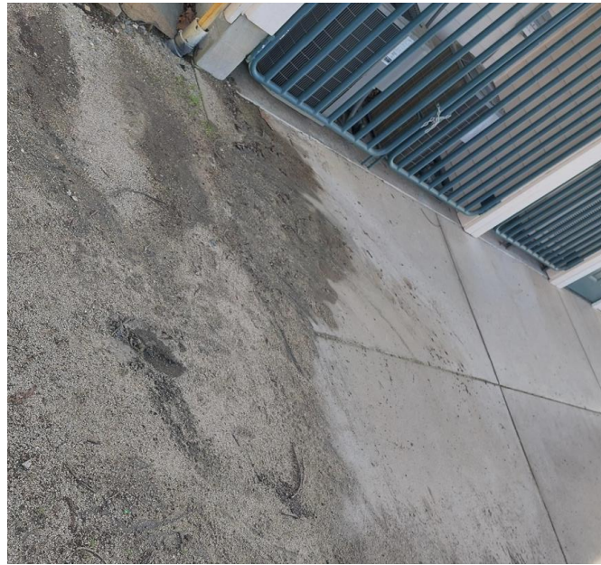
Figure 3: Erosion of DG around playground and behind Community Center
