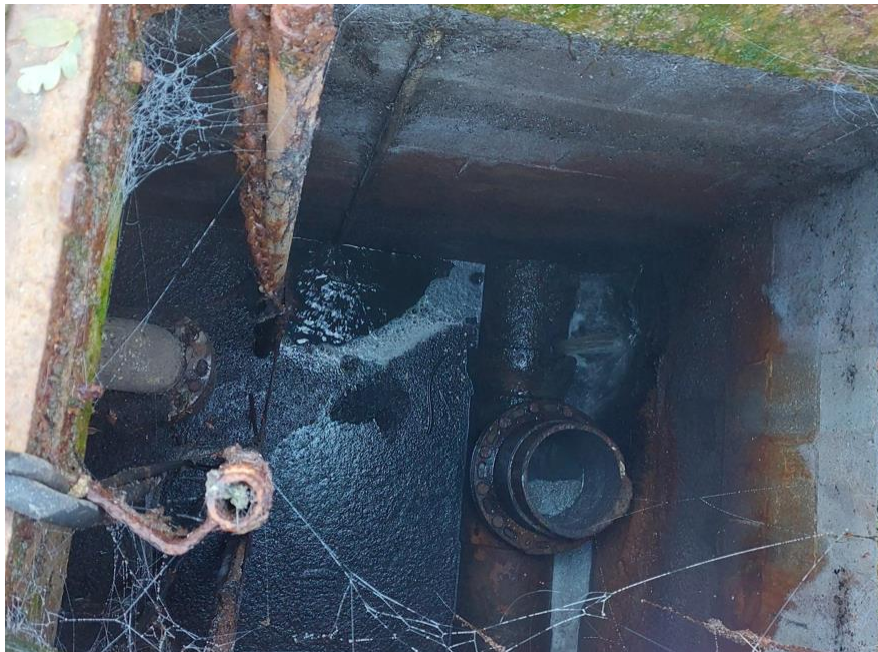
Return Valve in E-pump Vault
