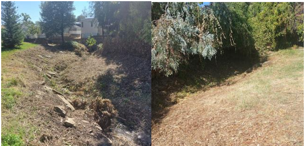
Bryson Drainage Ditch
