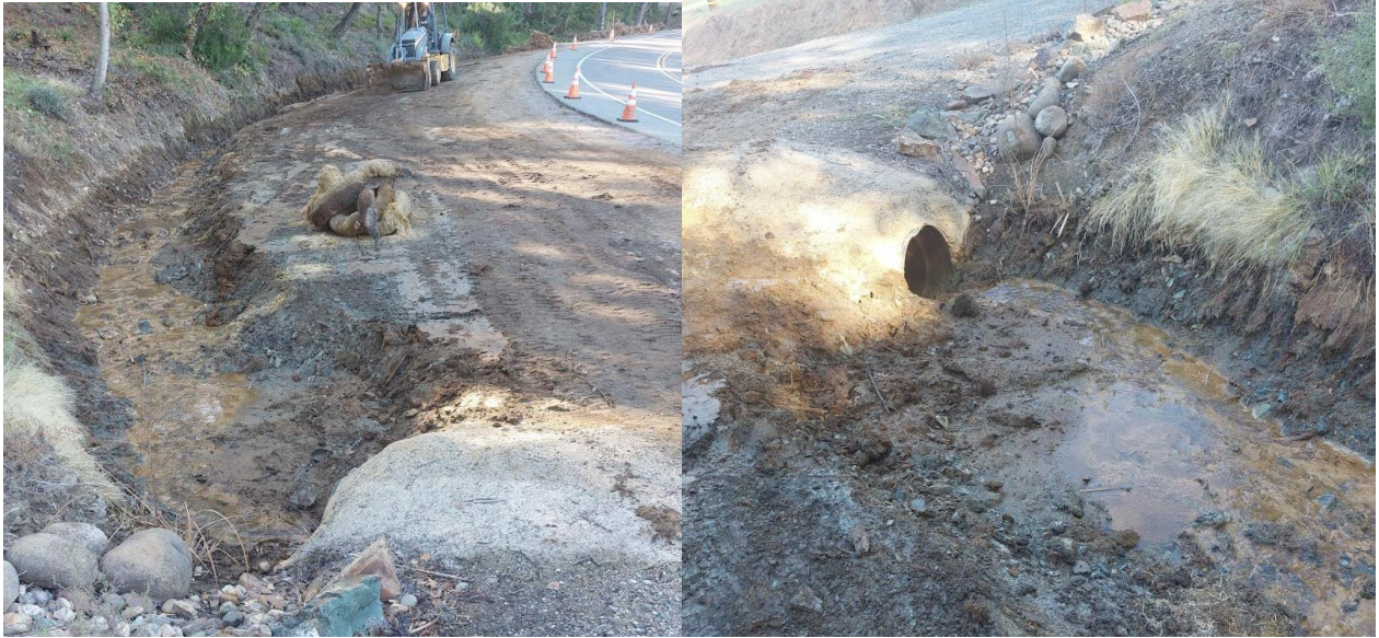
Miners Bend - Spoils removed (Drain pipe under Main Street cleared)
