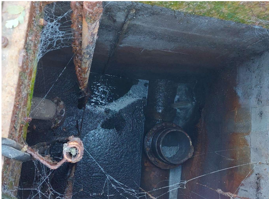
Return Valve in E-pump Vault
