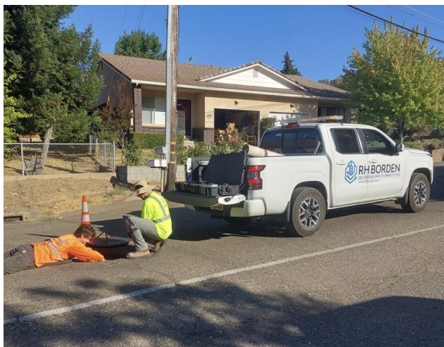
RH Borden Installing Flow Meters
