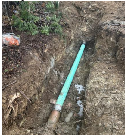
Repaired pipe (light blue)
