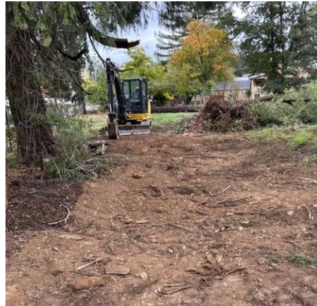
Finished repair to grade
