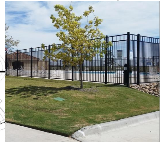
8' HT. ORNAMENTAL FENCE AROUND STADIUM – REPRESENTATIVE PHOTO
