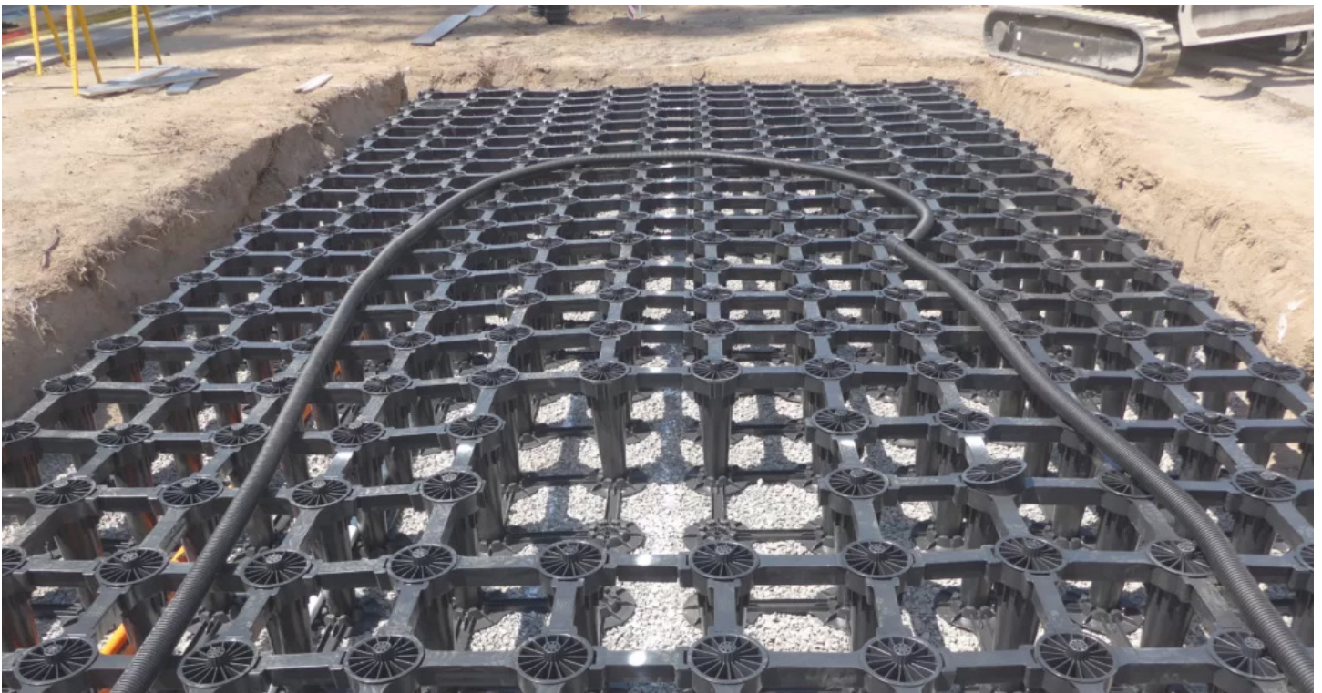
Green Infrastructure in Preparation for Site Development.
