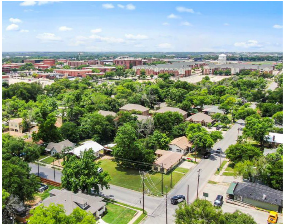
The residential neighborhoods in Stephenville are developed with a variety of housing types.
