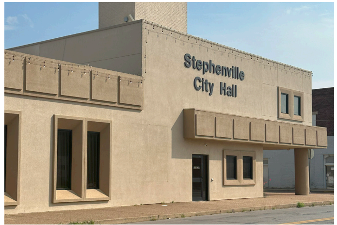
Stephenville's City Hall serves as the community's civic headquarters.
