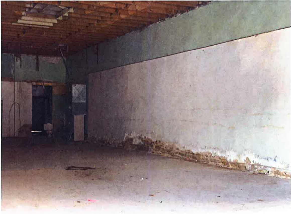
Figure 2 Interior North East Wall of Jake Wilson Building
