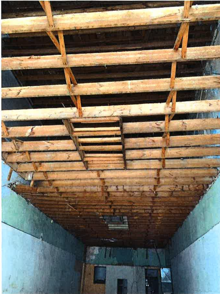
Figure 1 Ceiling of Jake Wilson Building Looking towards the North end of building with back facing Washington Street
