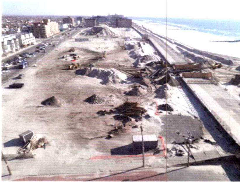
Sand Reclamation and Screening Site
