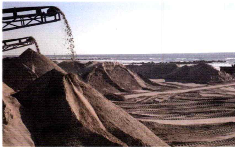
Clean Sand Coming Off the Screen onto the Beach
