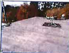
Flat roof view
