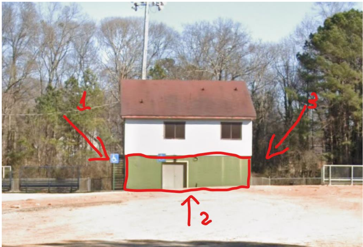
3 walls of the concession stand (the main wall facing the parking lot, and the two walls around).
