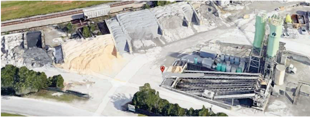
Exemplar: ready-mix concrete batch plant
