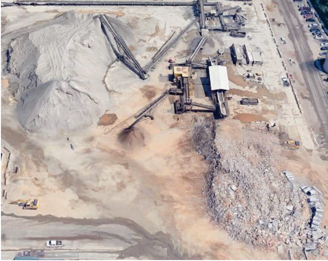
Exemplar: MetroGreen Pleasantdale concrete recycling facility
