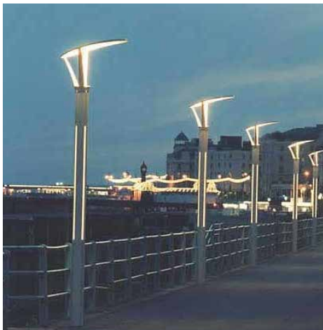
street lamps / lighting
