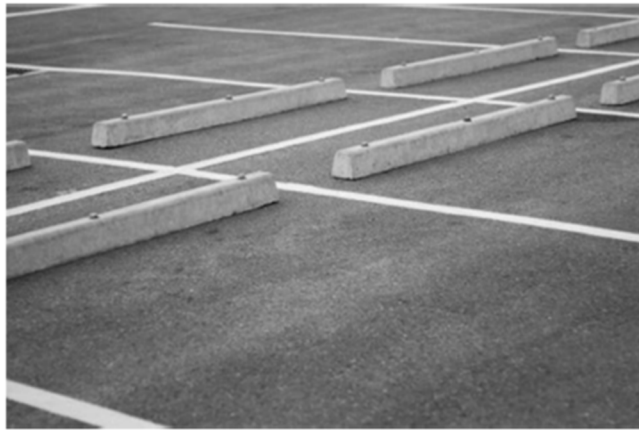
Wheel stop placement in "head-to-head" parking layout
