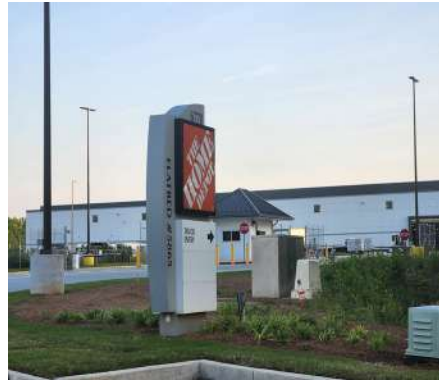
Caption: A logistics distribution center located in Stonecrest, GA
