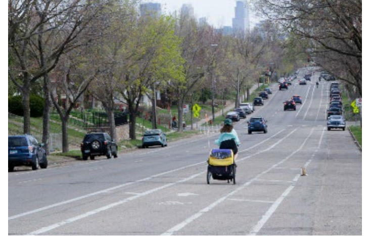
Painted Buffered Bike Lane (buffer can be on parked car side, travel lane side or both)
