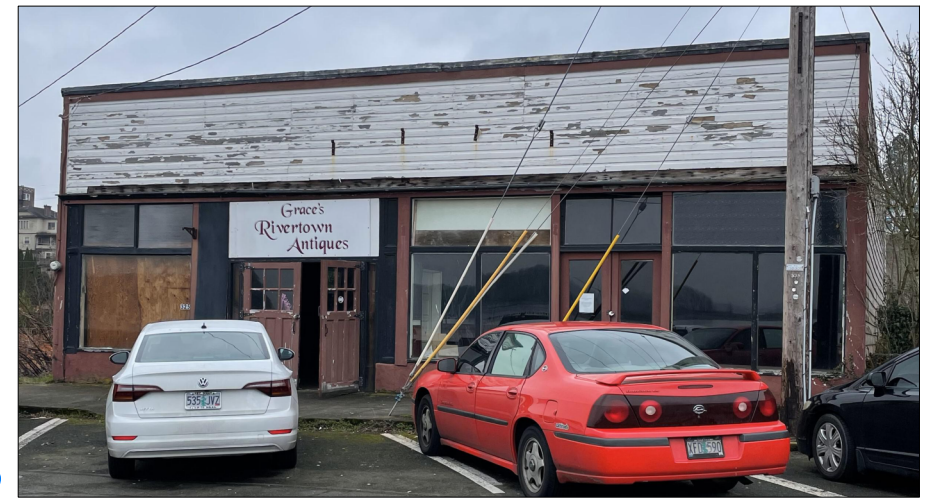
A VIEW LOOKING SE
