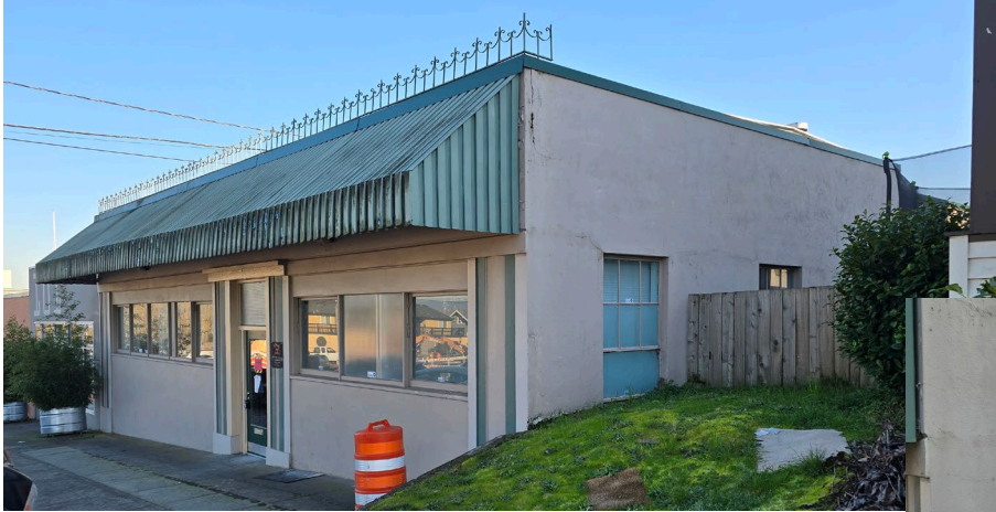
Left and Below: The west façade includes windows that face an abutting property developed with a dwelling.
