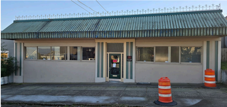
Left: Existing façade facing St. Helens Street. No modifications to this façade have been proposed to date.
