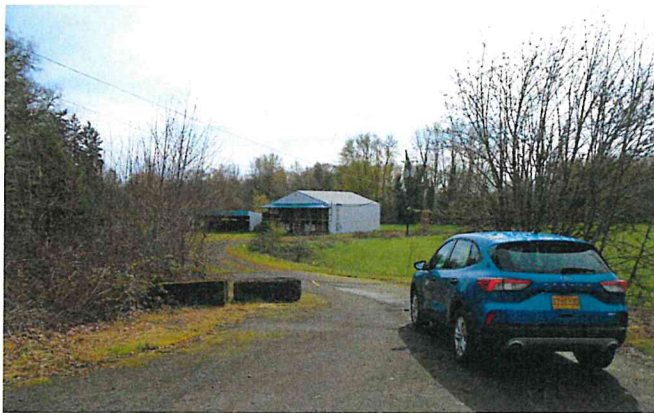
Subject property taken from Old Portland Road looking at access which is shared between property with existing buildings in the background and proposed new maintenance building (proposed on grassy field to the right of the existing buildings).
