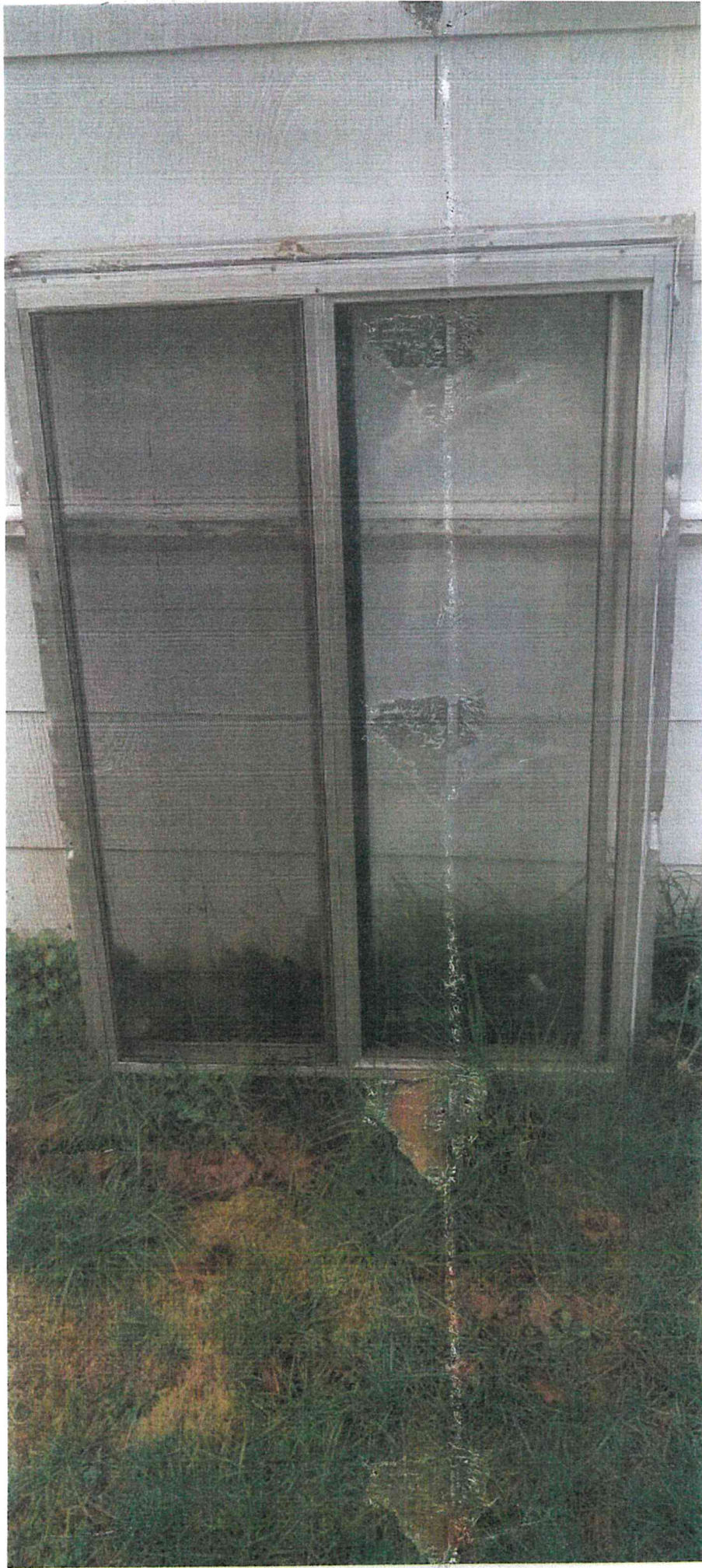
Aluminum Window Removed From North Elevation
