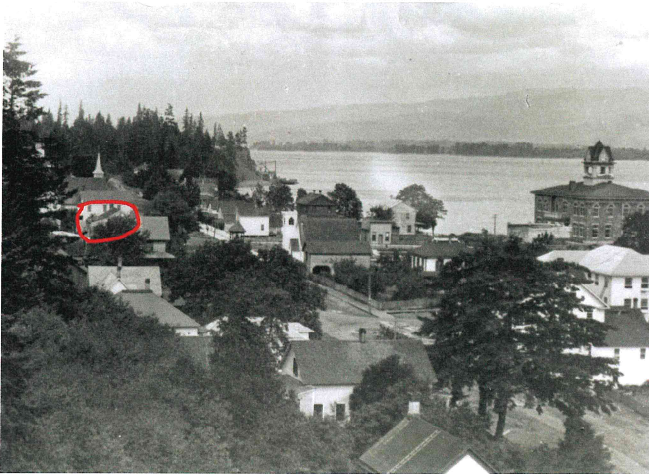
1909 - This appears to be the oldest photo of the structure. Photo courtesy CCMA.
