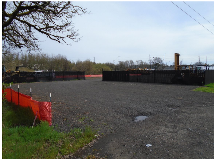
Photo taken March 29, 2024 looking northeast at the subject property from Gable Road.
