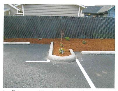
Approved plans showed an island width between curbs of 9' and a depth of 12' as measured from the landscape edge on the right side as seen in this photo (i.e., the short edge). Instead of the 9' x 12' dimension of the approved plan, this island was installed as 3' x 4' including the curb.
