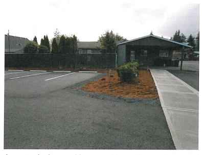
Approved plans had this area at 17' between the sidewalk and curb. It also showed a curb on the opposite side of the sidewalk. It was only constructed with an approximate 13' length between the back of sidewalk and parking stall. No curb was installed. In addition, a street tree was installed with a dba of much less than the normal 2" minimum.
