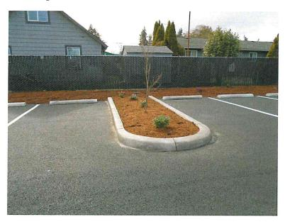
Approved plans showed an island width between curbs of 7 feet. It was constructed at 5' between the curbs. The minimum width is 6' between curbs. Being slightly off from the minimum and having a tree that more closely honored the 2" caliper identified on the approved plans, this is the least problematic of the three islands and is a fair representation of a typical landscape island not along a street.
