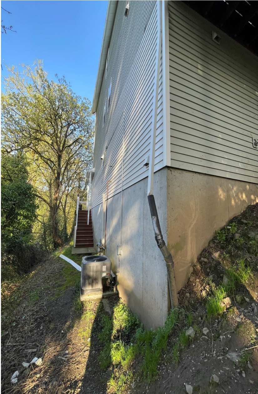
Use of 10-foot stem wall contoured to topography
