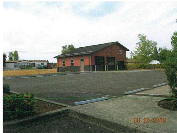
Subject property's parking lot and garage/storage building
