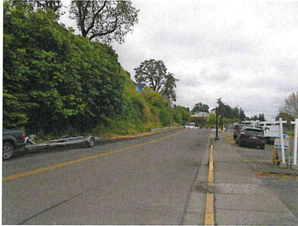
River Street roadway looking north
