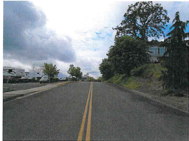
River Street roadway looking south
