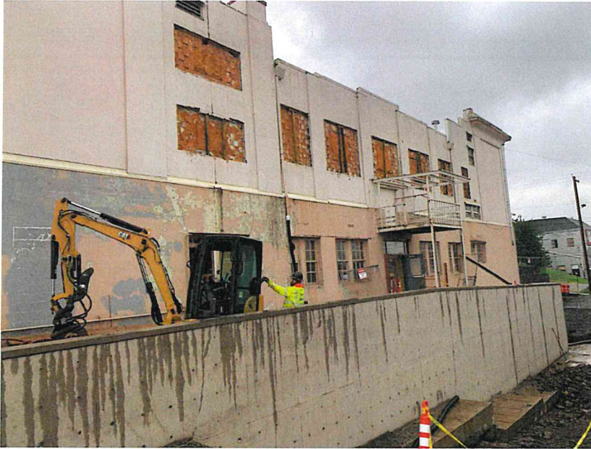
2A. View from SW during construction showing full facade
