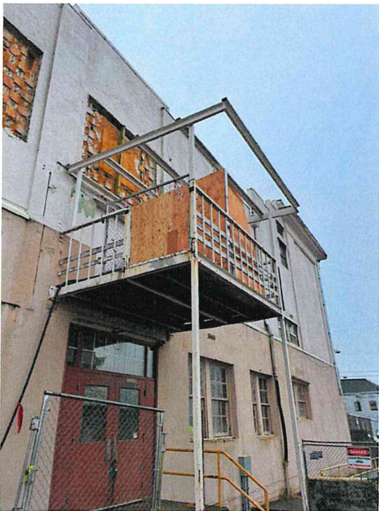
1B. View from SW during construction showing close-up of porch
