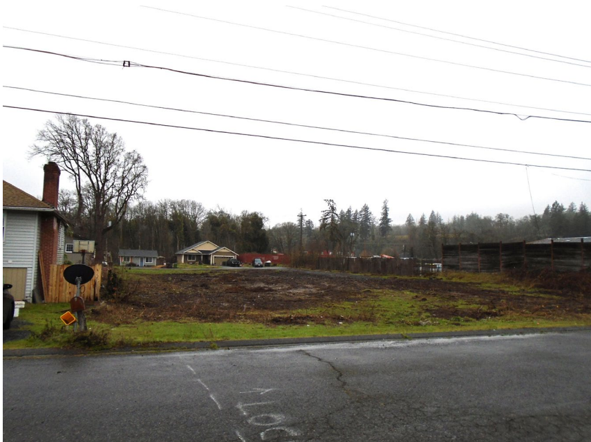
Above left: Subject property in March 2023 after it was cleared. This photo taken from N. 12 th Street. The fence/wall that surrounded the former mill site is visible to the right of the photo.
