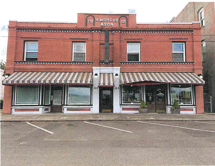
Left: Morgus building adjacent to subject property on Strand Street demonstrating storefront window kickplates/paneled bulkheads
