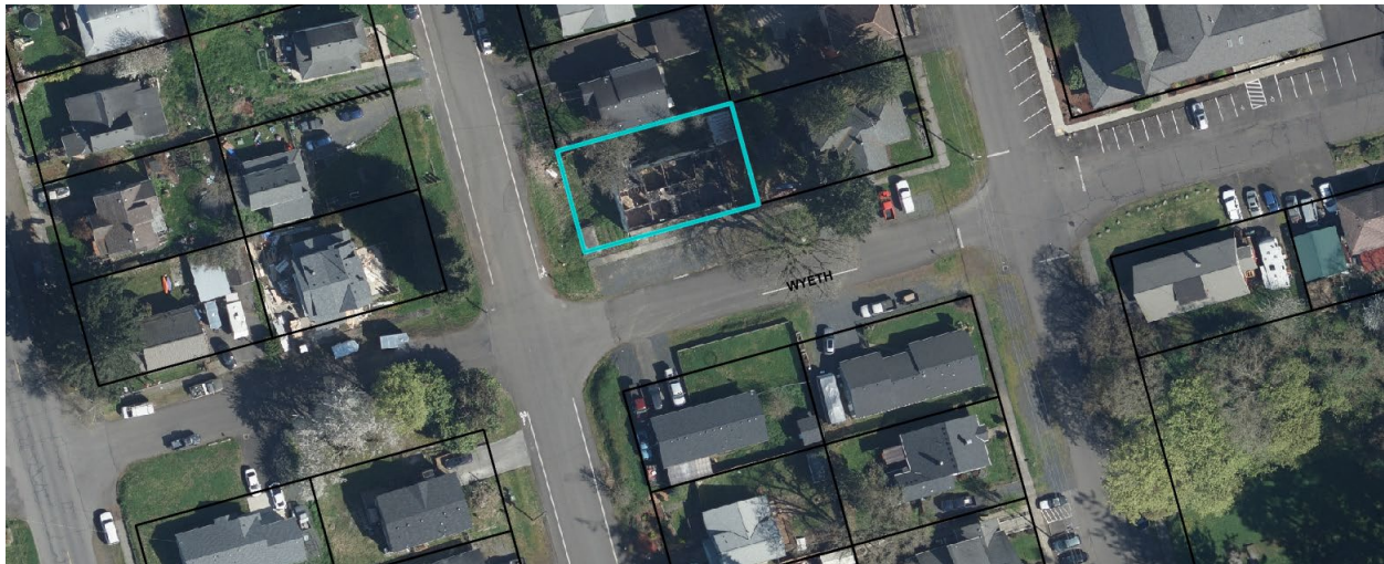
Above: April 2022 aerial photo with the subject property outlined in blue. The back lines are property or right-of-way lines. Note the proximity of other buildings along the north side of Wyeth Street.
