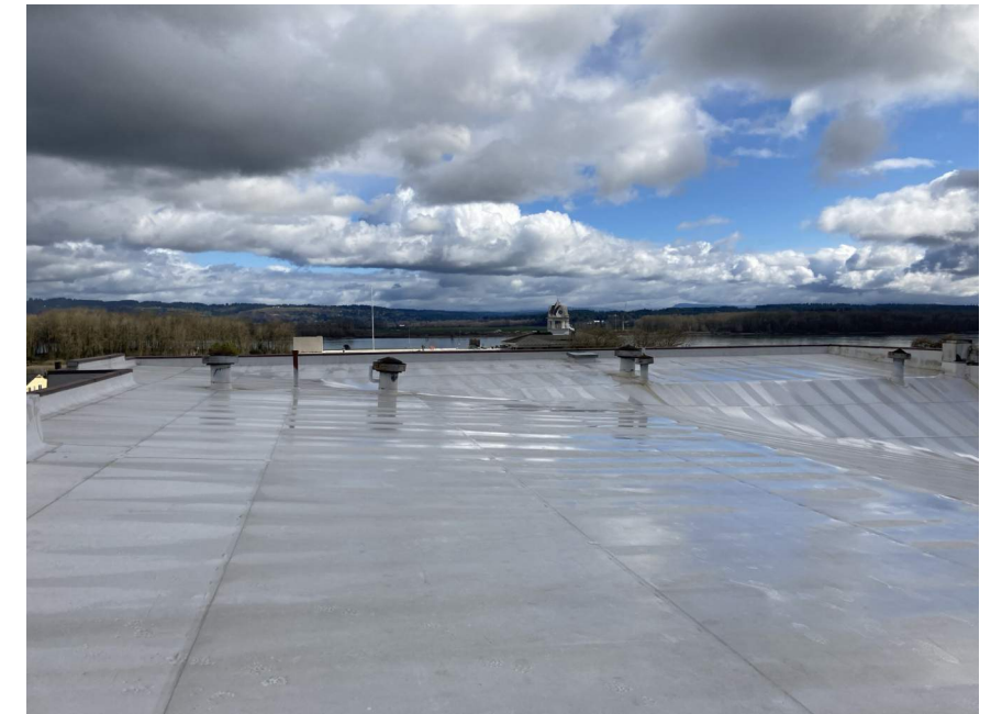
06 VIEW OF ROOF
