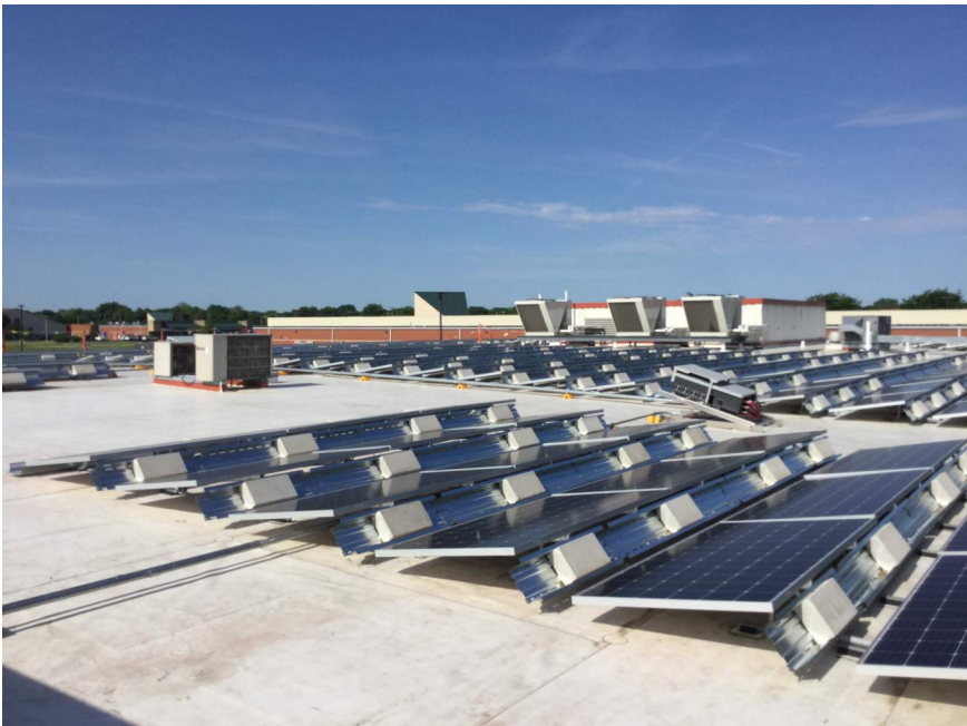
EXAMPLE IMAGE: BALLASTED PHOTOVOLTAIC PANELS & INVERTER ROOFTOP INSTALLATION
