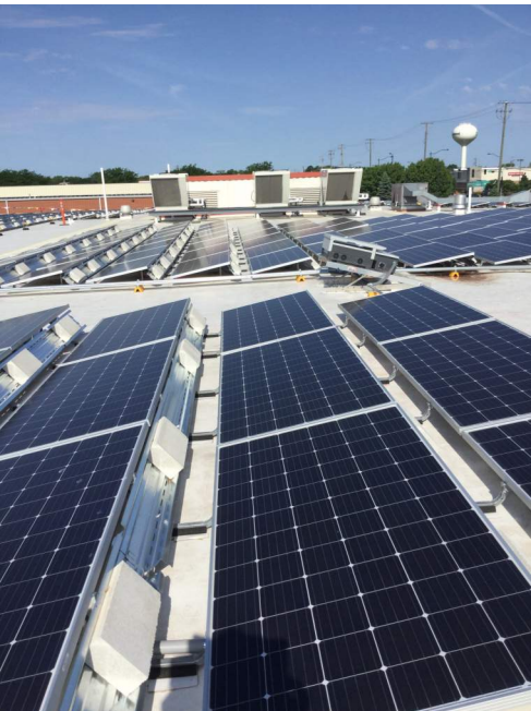
EXAMPLE IMAGE: BALLASTED PHOTOVOLTAIC PANELS & INVERTER ROOFTOP INSTALLATION
