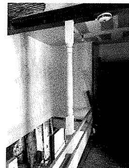
Existing interior structural turned post that we will match for porch posts.
