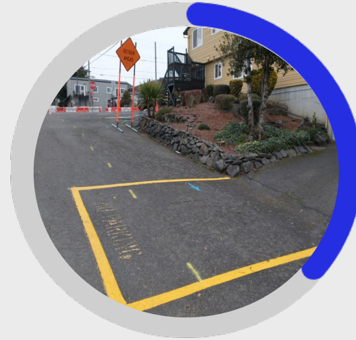
S 1 st St/St. Helens St Undergrounding
