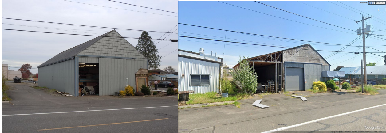
Left Photo: February 10, 2014 of 184 S. 15 th Street before the proposed building addition. Right Photo: Google Earth street view May 2023 long after the building addition project had been abandoned and permits expired, but landscaping was still intact, including the area between the building and sidewalk. This shows a driveway along the north side of the building that was eliminated with the building addition.
