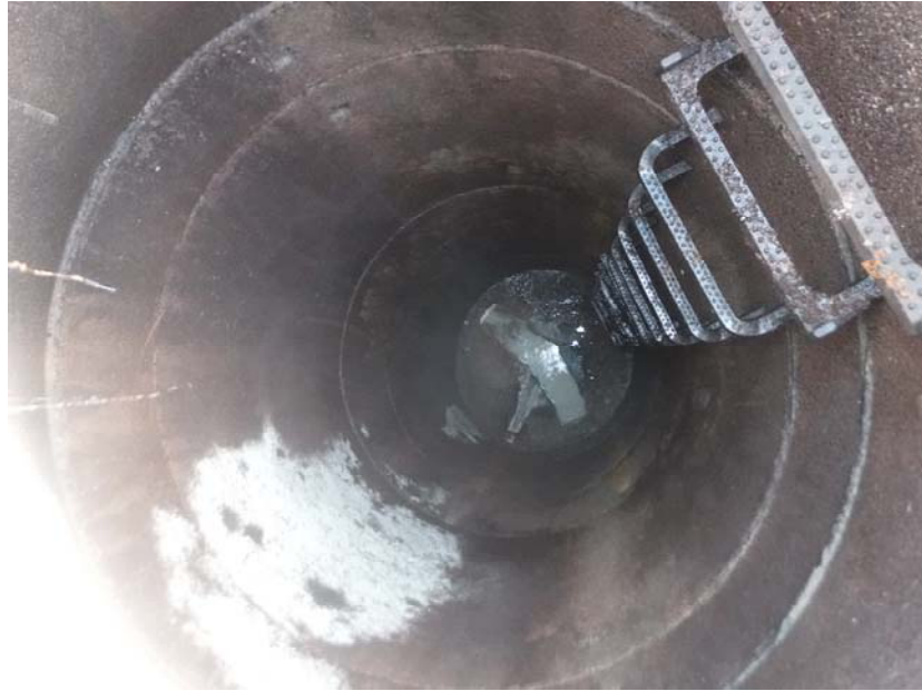
Figure 4. Skamania Lodge discharge manhole sampling location.
