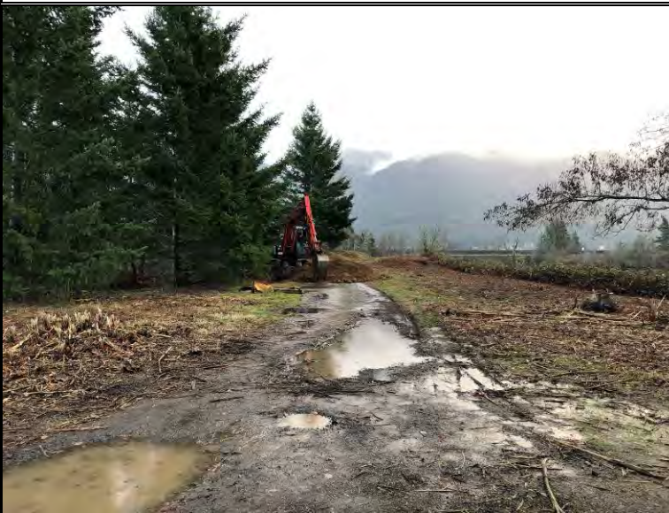
Excavation of test-pit TP-12, looking southwest
