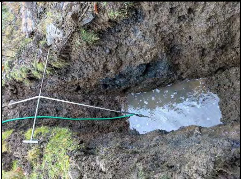
Infiltration test setup at test-pit P-1
