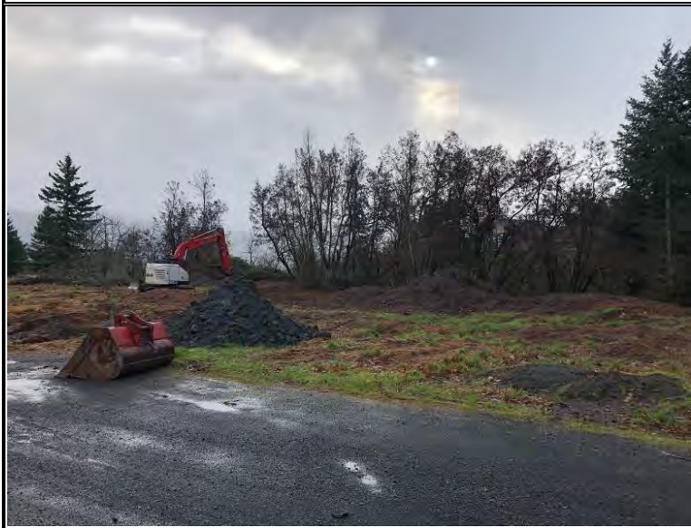
Excavation of test-pit TP-2, looking southwest
