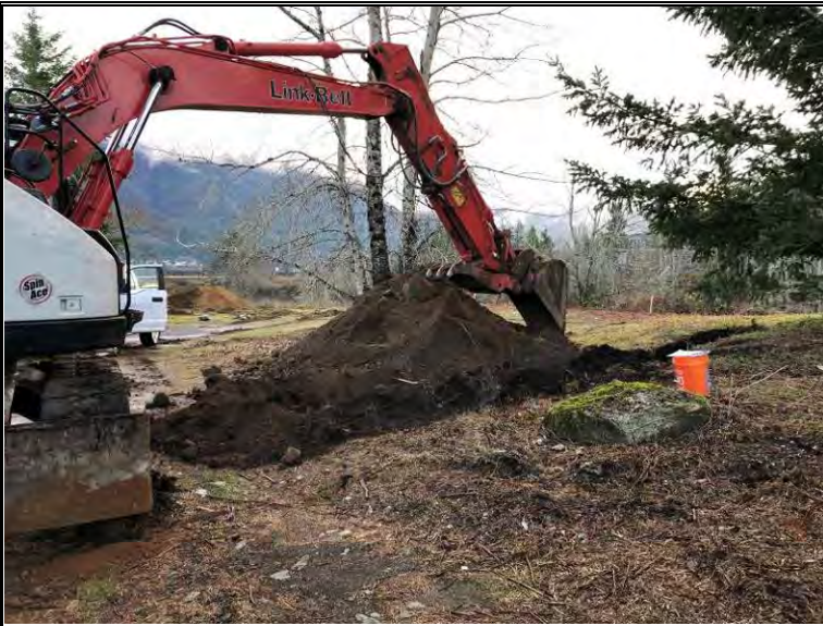
Exposed subsurface soil profile within test-pit TP-11
