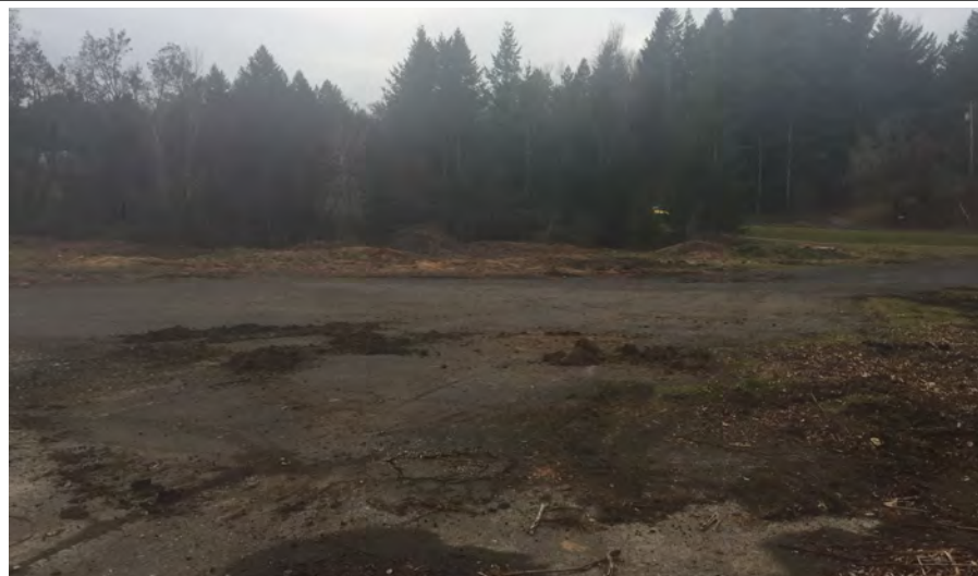
Photo 2. Existing concrete and gravel surfacing.
