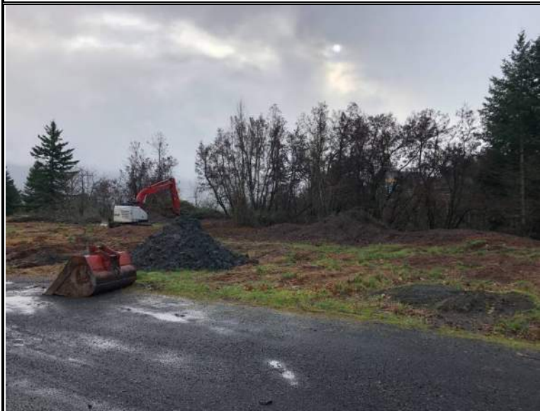
Excavation of test-pit TP-2, looking southwest
