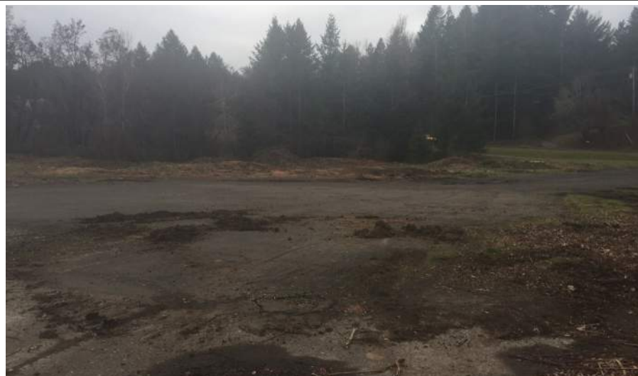
Photo 2. Existing concrete and gravel surfacing.
