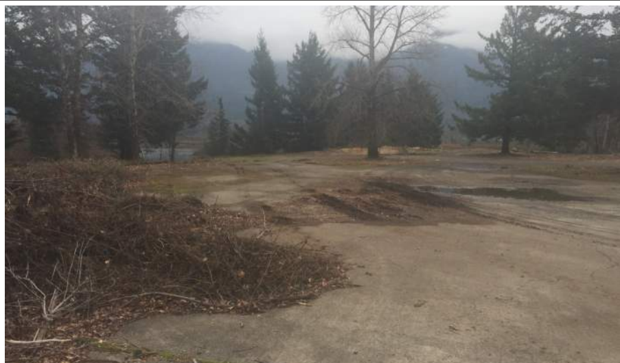
Photo 1. Existing concrete and gravel surfacing.
