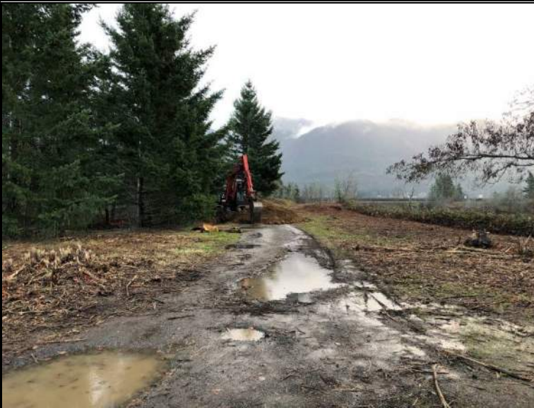
Excavation of test-pit TP-12, looking southwest
