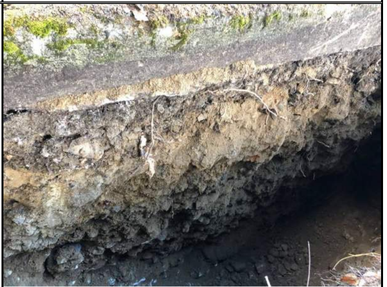
Exposed subsurface soil profile within test-pit TP-6
