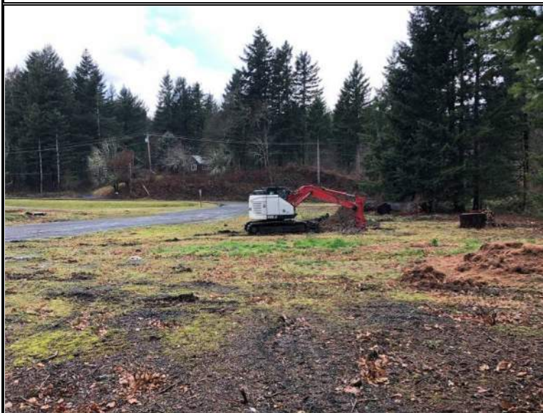
Excavation of test-pit TP-3, looking west
