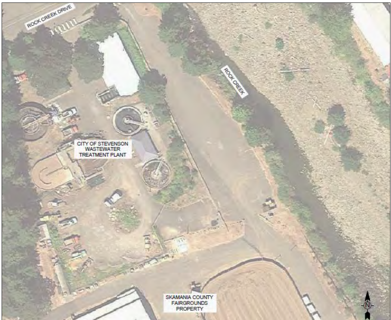
Figure 6-1. Stevenson WWTP Site
