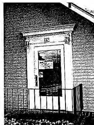
Appropriate: Wooden door frame with wood detailing above
