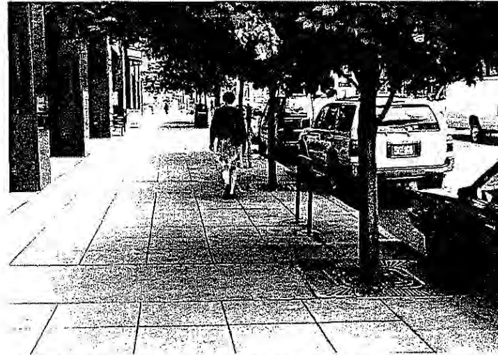
Appropriate: Gridded concrete sidewalk with street trees in square grates and a bike rack
