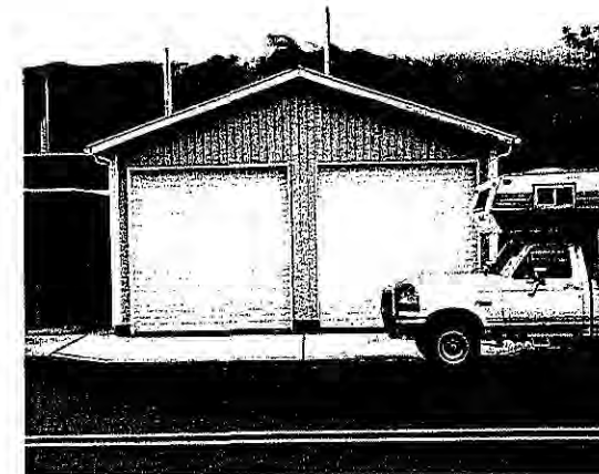
Not Appropriate: Overhead Garage doors engaging public streets
