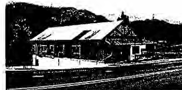
Appropriate: One-story wood frame building
