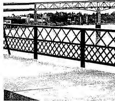
Appropriate: Lace-like Steel balustrade
