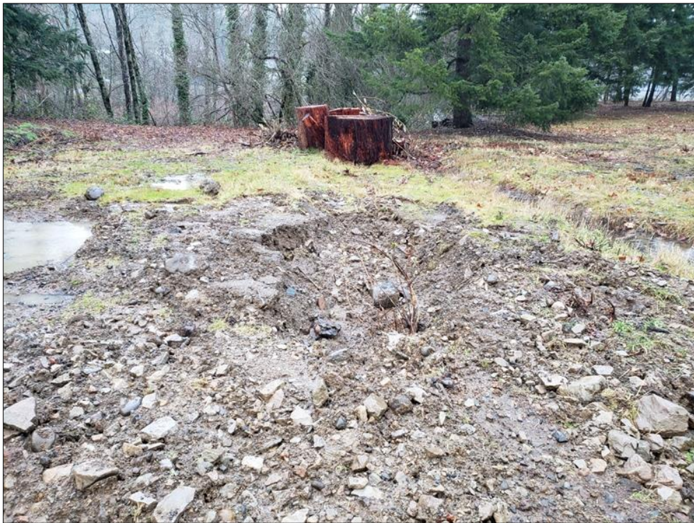
Figure 5. Photographic overview looking northeast of an area that had been trenched prior to fieldwork.
