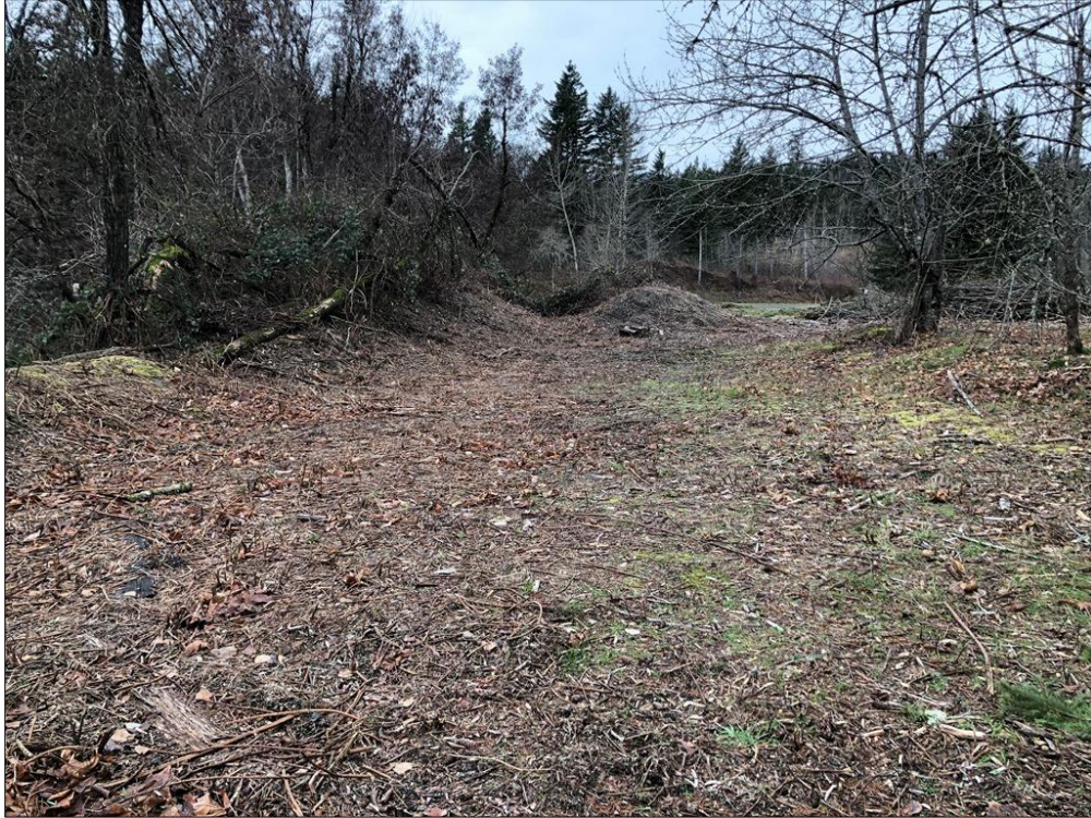
Figure 4. Photographic overview looking north of an area cleared of brush. The vegetation and displaced soil have been pushed into low piles.
