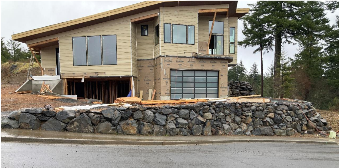
Figure 2 – 725 Angel Heights Rock Wall Looking East
