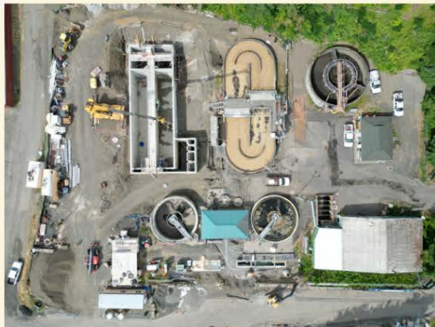
Stevenson Wastewater Treatment Plant
