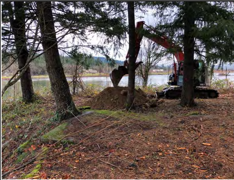
Excavation of test-pit TP-5, looking east
