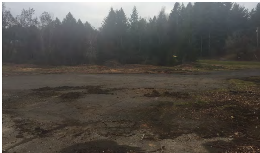
Photo 2. Existing concrete and gravel surfacing.
