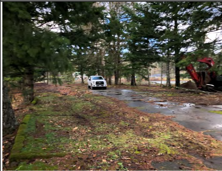
Excavation of test-pit TP-6, looking north
