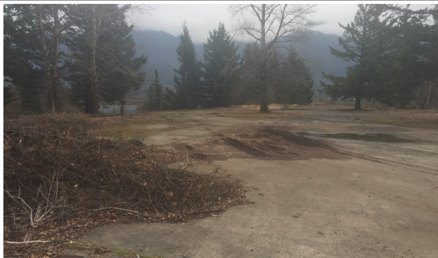
Photo 1. Existing concrete and gravel surfacing.
