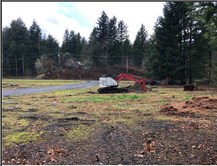
Excavation of test-pit TP-3, looking west
