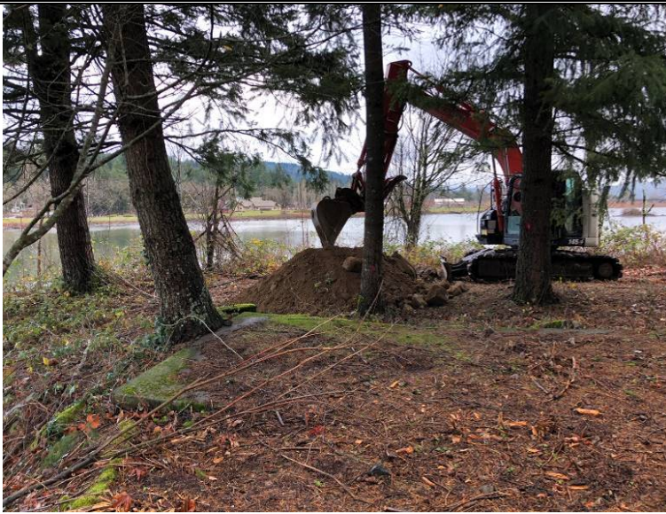
Excavation of test-pit TP-5, looking east
