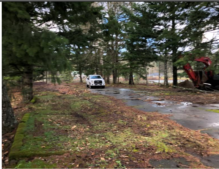
Excavation of test-pit TP-6, looking north
