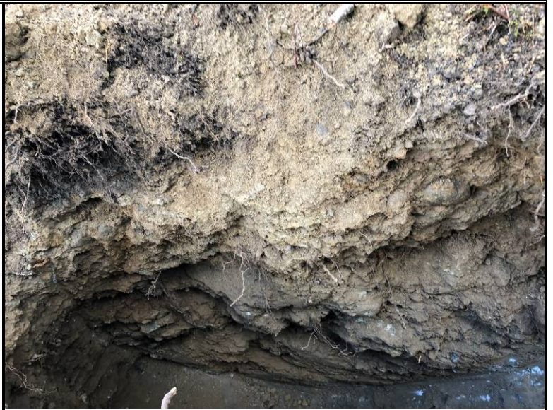
Exposed subsurface soil profile within test-pit TP-5
