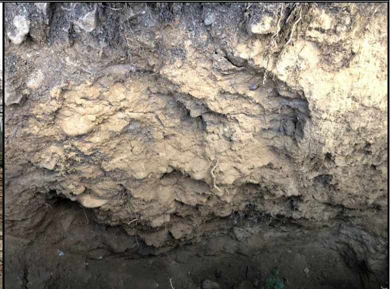
Exposed subsurface soil profile within test-pit TP-12
