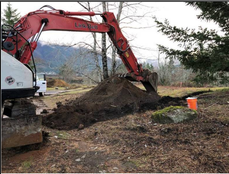
Exposed subsurface soil profile within test-pit TP-11
