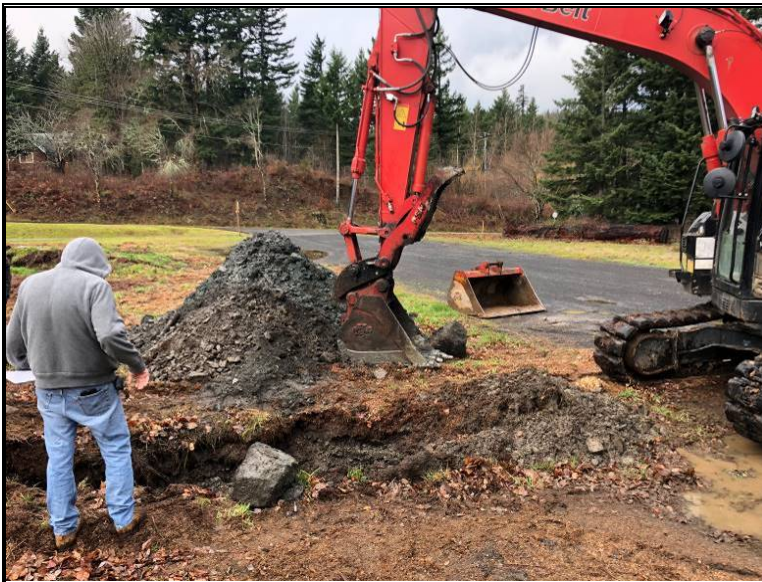
Excavation of test-pit TP-1, looking west
