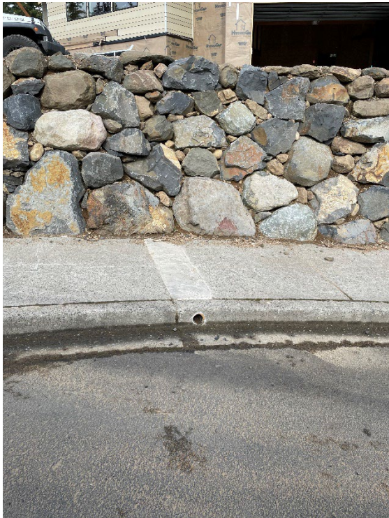
Figure 5 - Sidewalk Cut for Wall Drain
