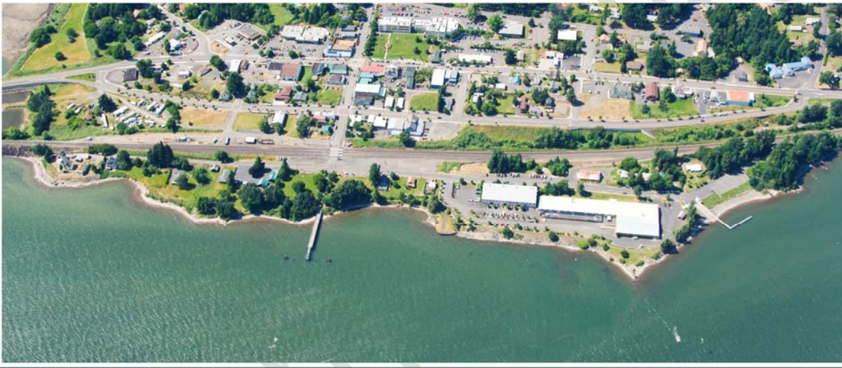
Figure 4.2-1 Columbia River Reach 2 Downtown Stevenson's urbanized waterfront area
