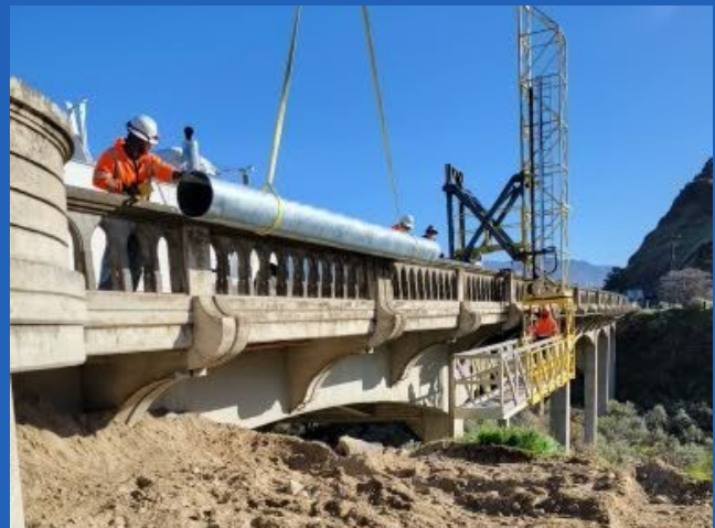
Water line installation under the bridge. Photo credit: Anderson Perry
