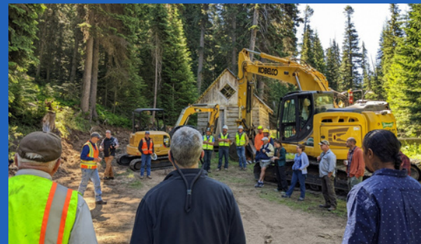
Ground breaking at the Dog River water pipeline replacement
