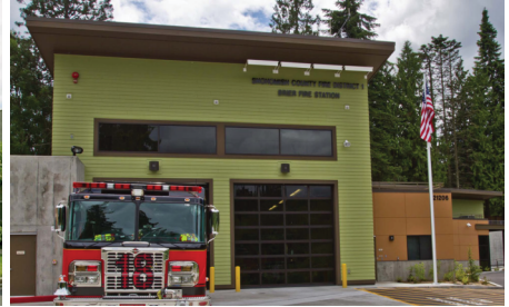
A5 Snohomish County Fire Station 18 - TCA
