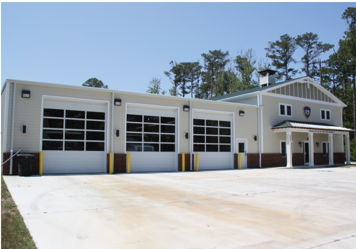
Roanoke Island Fire Department PREMIERE CONTRACTING
