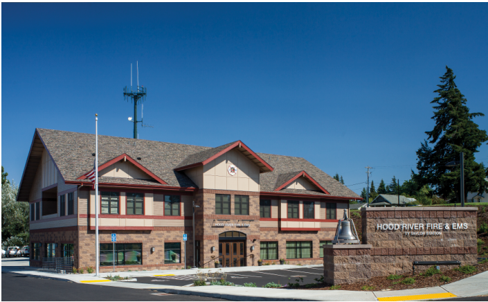
Hood River Fire Station MACKENZIE
