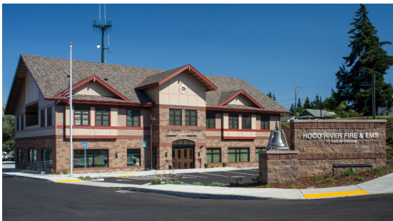
Hood River Fire Station - Mackenzie
