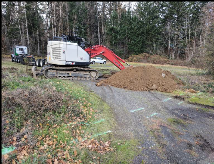
Excavation of test-pit TP-2 looking south
